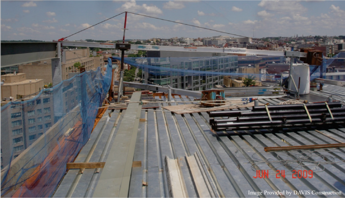
Image Provided by DAVIS Construction
